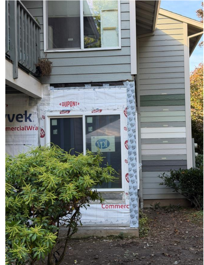
Woodspring Apartments Renovation, Tigard, OR
