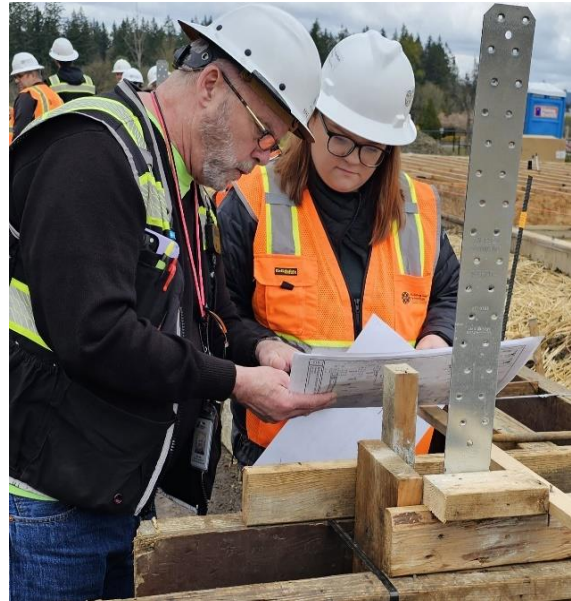
Inspector Mike Ditty & Student Haylie Black Performing a Foundation Inspection
