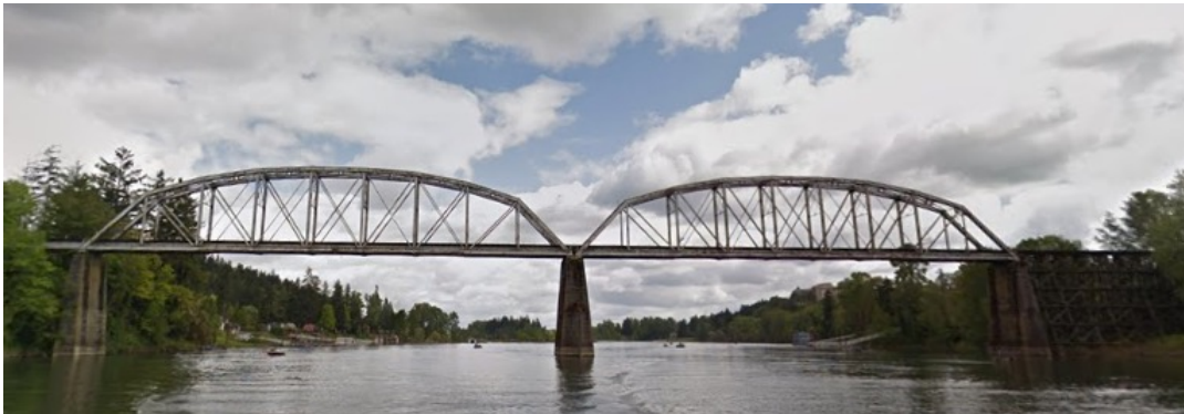
Oak Grove – Lake Oswego Railroad Bridge
