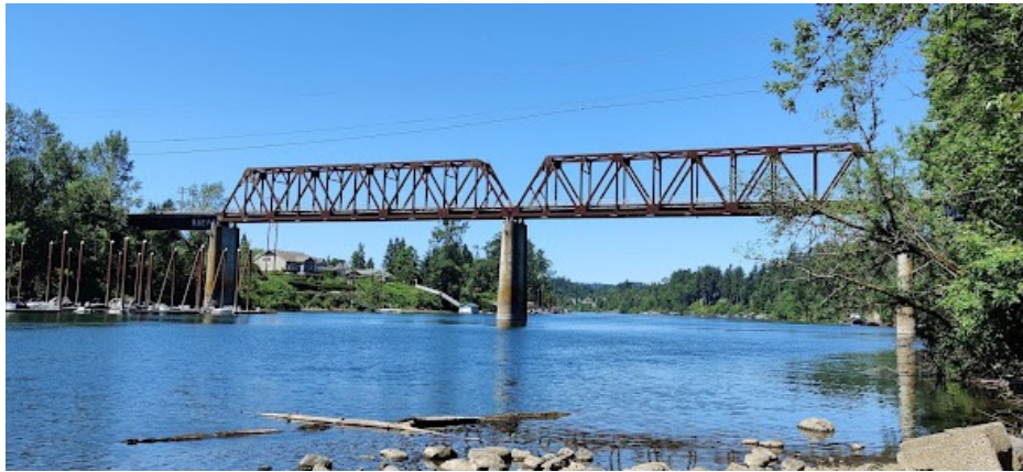
Willamette Rail Bridge - Wilsonville
