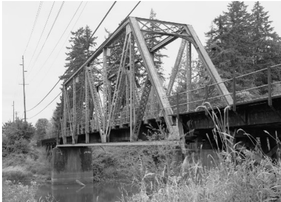
Tualatin Railroad Bridge – Milepost 35.3
