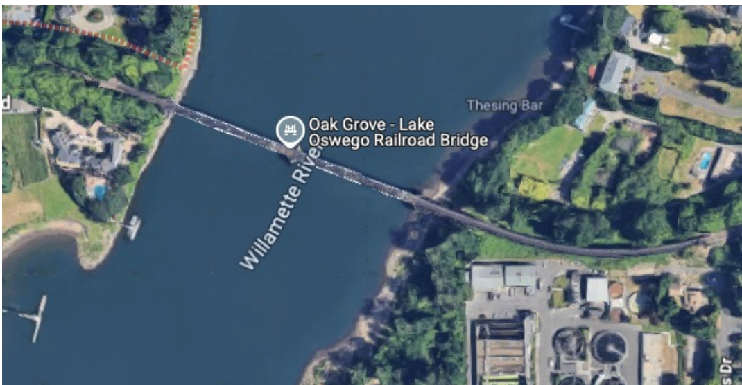
1910 Portland and Western Railroad Cascadia threat discovered 2010
