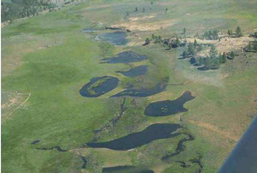
Figure 1: Post-project aerial photo of Last Chance Creek (2005). The series of ponds and plugs mark the location of the pre-project gully. The widths of constructed plugs indicate pre-project gully width. Historic remnant channels are used for the base flow channel of the restored system. (Photo: Jim Wilcox)
