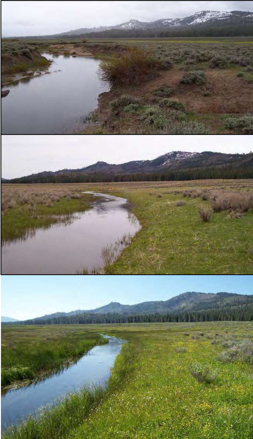
Figure 2: Pre- and post-project photos of the 2006 Red Clover–McReynolds Project (2006, 2007 and 2008). The pre-project gully is more than 10 feet deep and 90 feet wide. The steep gully banks are actively eroding. Erosive flood flows for the post-project channel easily access the meadow’s broad floodplain, drastically reducing shear stress and resulting in stable stream banks (middle photo, 2007). The bright green vegetation line in the pre-project photo (upper right) is the location of the post-project base flow channel. The bottom photo (2008) shows vigorous riparian vegetation recovery on the channel banks and a narrowing of the channel due to capture of fine sediments. The narrower and deeper channel should result in cooler stream temperatures. (Photos: Jim Wilcox)
