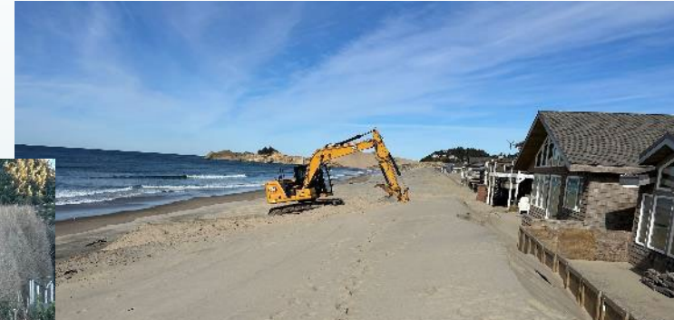
Remedial grading where there is approved management plan and sand is inundating homes
