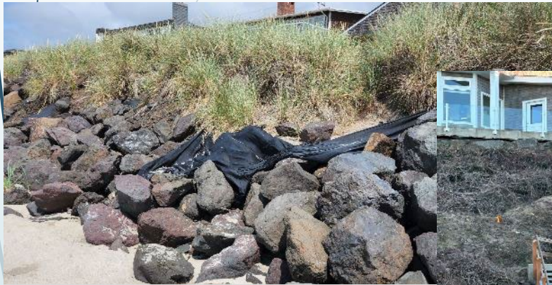
Maintenance of permitted structures
