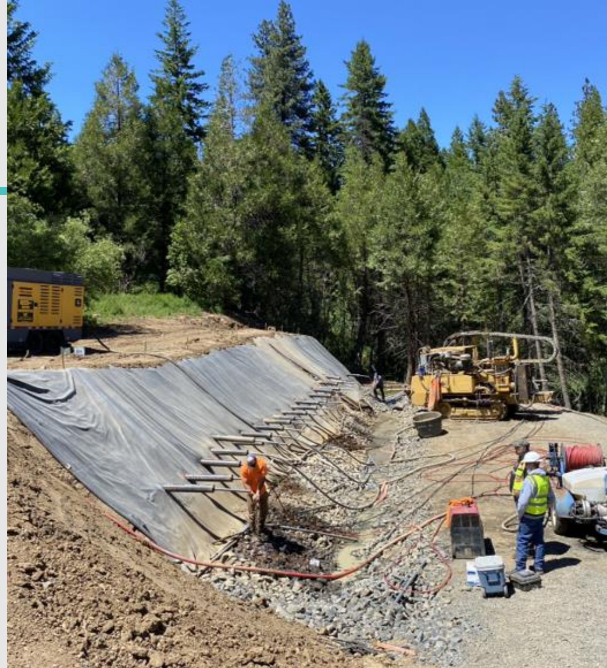
Unstable slope mitigation under construction for seismic resiliency on I-5 at Siskiyou Station (MP 5.2, ODOT Region 3)
