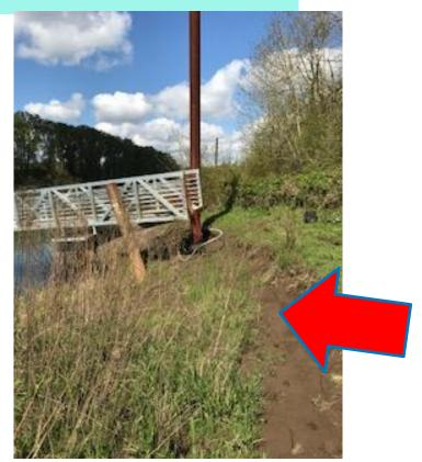
This land (30 feet) has now almost completely eroded. In prior years, this land would flood during winter/spring, but there was no riverbank erosion as illustrated in the next slide. Gangway had to be lowered 3 feet & additional ramp had to be added to gangway for access.
