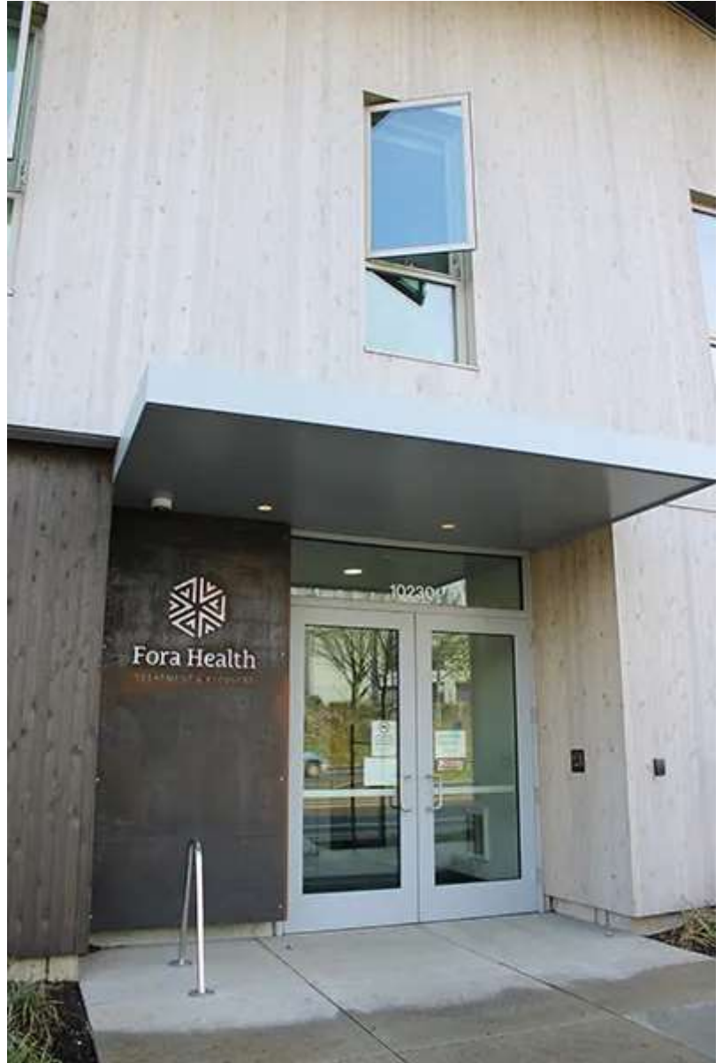
$4.5 million in public funds went into constructing DePaul Treatment Center, now Fora Health. That meant workers were supposed to be paid prevailing wage. But drywall workers had trouble being paid at all.
