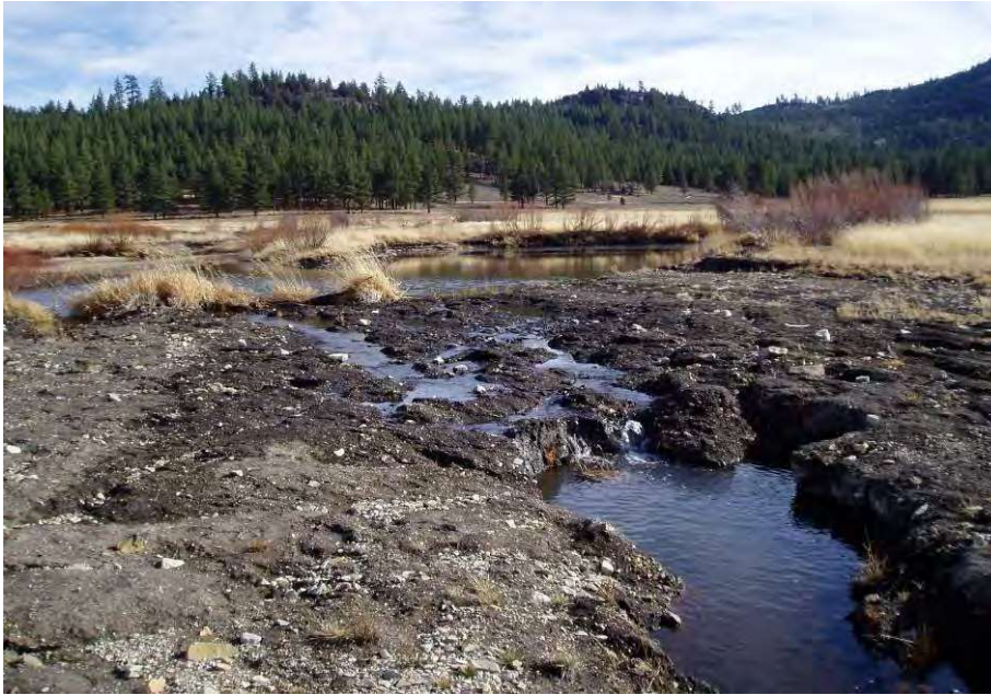
Figure 11: Excessive flow over this plug on Last Chance Creek at Jordan Flat during the 2006 floods caused the base flow to be diverted over the plug. Excessive flow was due to unforeseen dynamics between Last Chance Creek and a tributary stream. A berm was constructed and the problem corrected in 2007. Excessive flow over plugs could headcut through the entire plug, lowering the upstream pond elevation to the elevation of the downstream pond and essentially doubling the head on the next upstream plug. (Photo: Joe Hoffman)
