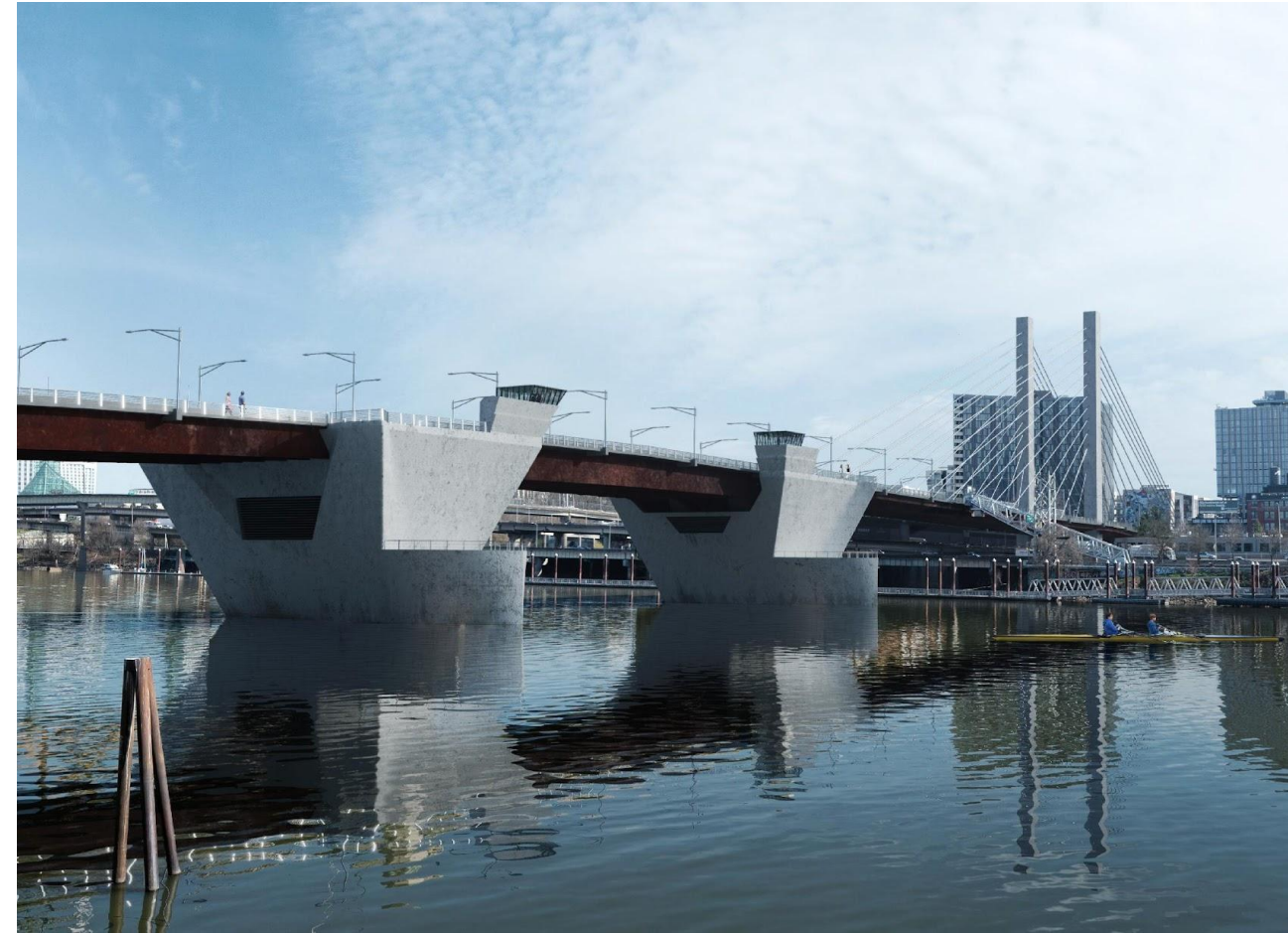
with Cable Stay Tower
