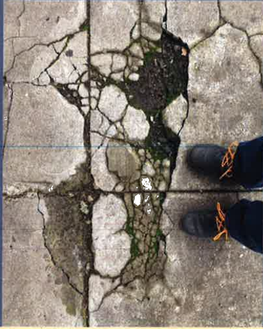
Example of Third Street sidewalk cracks
