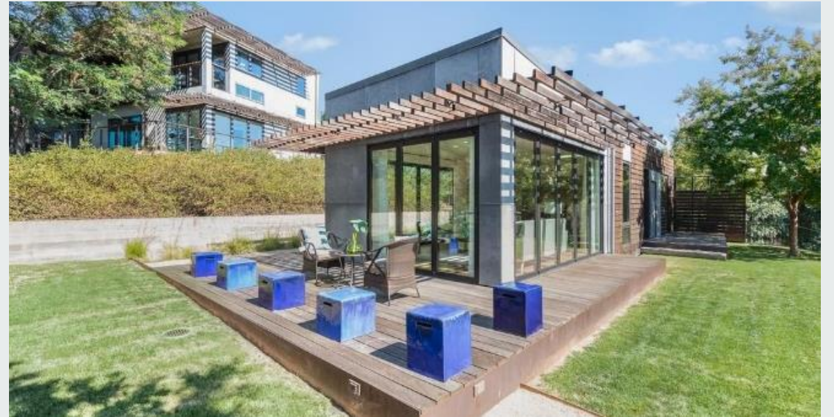
Taylor House, San Francisco (2009) ADU + Main house
