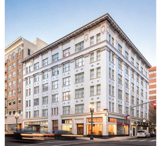
Central City Concern's Henry Building, located at SW 4 th and Oak in Portland, underwent a major seismic renovation and preservation completed in 2021. Colas Construction was the project's General Contractor.
