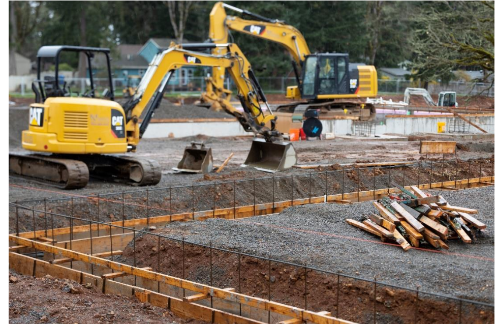
Groundbreaking: Mahonia Crossing
