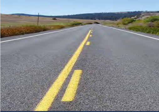
Good Pavement Conditions
