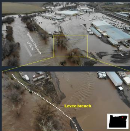
Images taken from video from: City of Pendleton, 2020. Umatilla Flood I84 to Reith.
