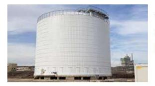
Typical large liquid **ammonia** store **312,000 MWh** (60,000 tonnes @ -33°C)
