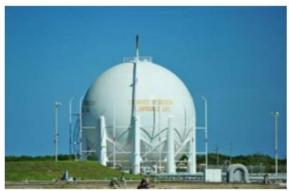
World's largest liquid **hydrogen** store Cape Canaveral **9,000 MWh** (270 tonnes @ -253°C)
