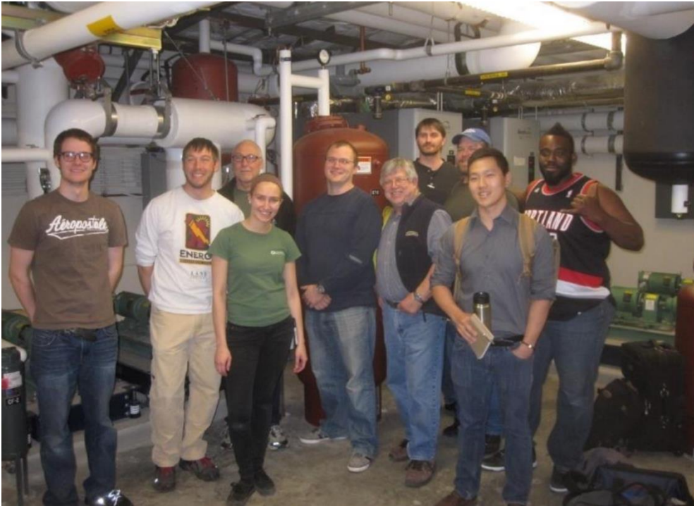
Building Energy Controls Apprenticeship Program at Lane Community College
