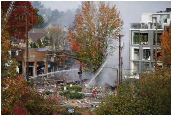
A natural gas explosion in NW Portland in 2016 damaged a city block.
