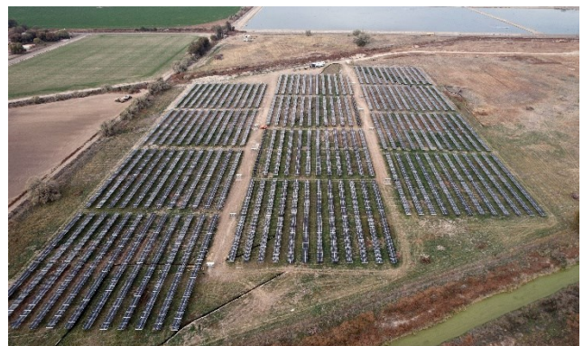
The City of Ontario's Verde Light Oregon Community Solar project was the first completed Community Renewable Energy Grant-supported project.
