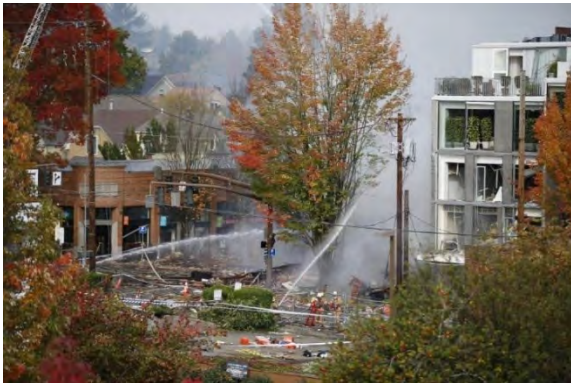
A natural gas explosion in NW Portland in 2016 damaged a city block.
