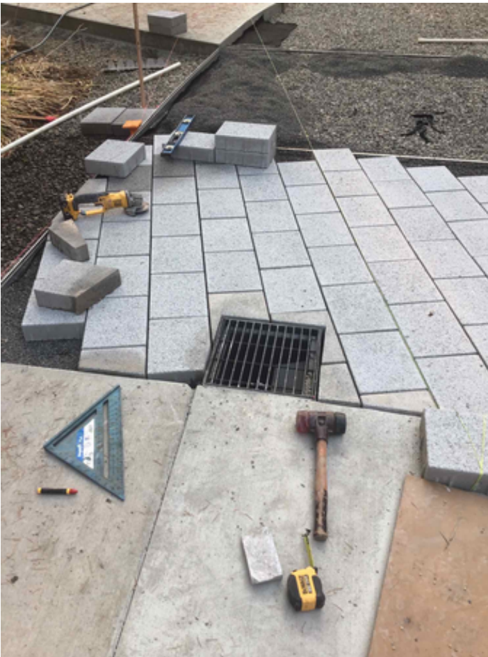
Paver Installation
