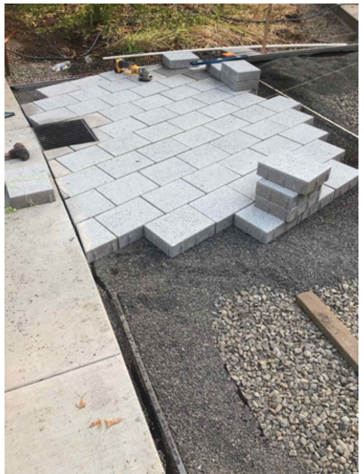
Paver Installation
