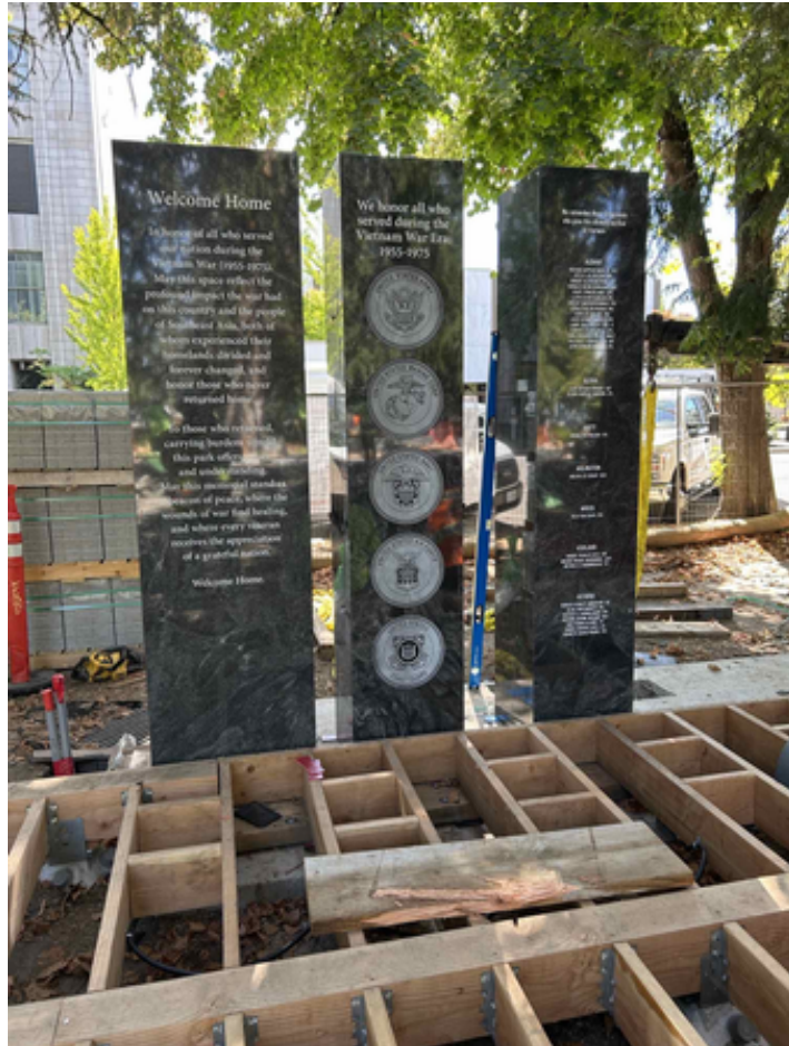
Granite Column Install 9/9/2024
