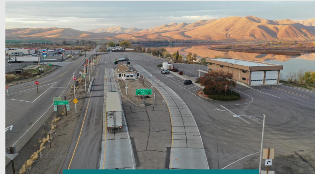
Farewell Bend Point of Entry Station
