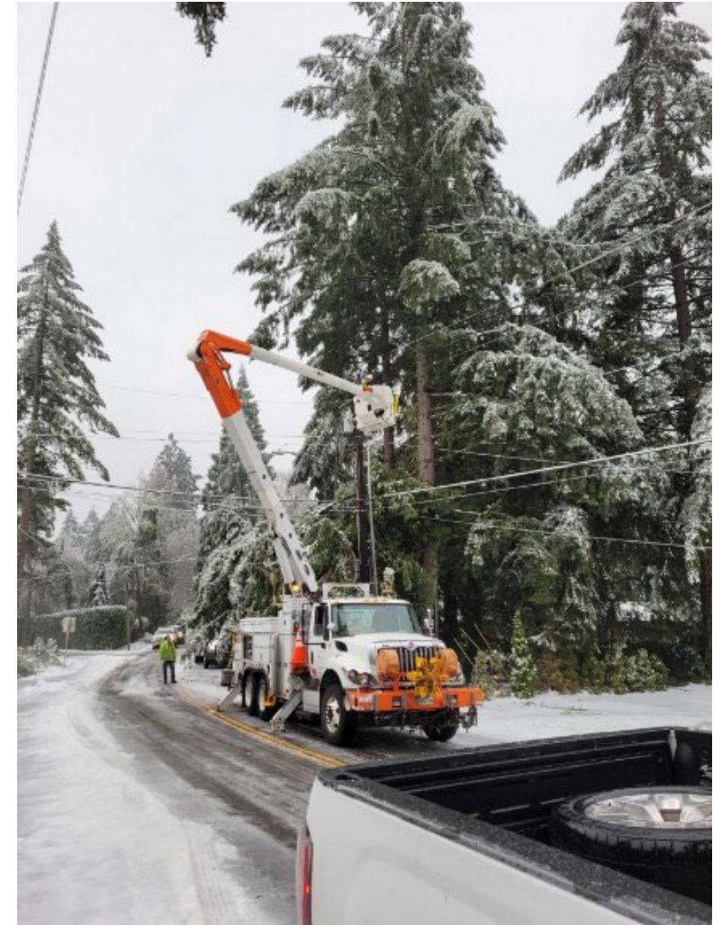
Figure: Crews working in Icy Road Conditions
