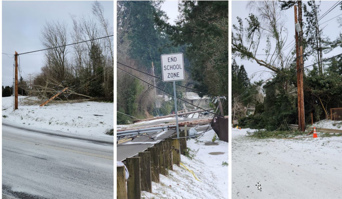
Figure 1: Photos of Extensive Damage and Hazardous Road Conditions
