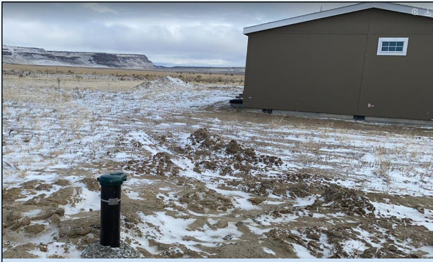
Domestic Well in Eastern Oregon
