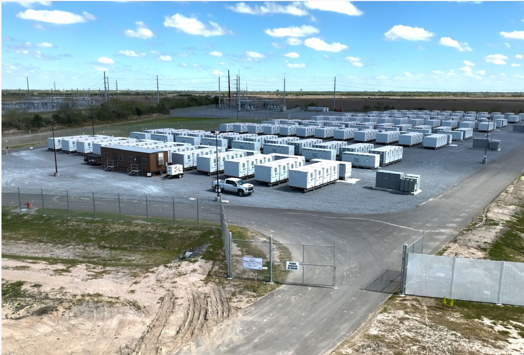
Aerial photographs of Eolian, L.P.'s Madero & Ignacio battery energy storage facility, a 200 MW/2.5+ hour duration storage system in Texas.
