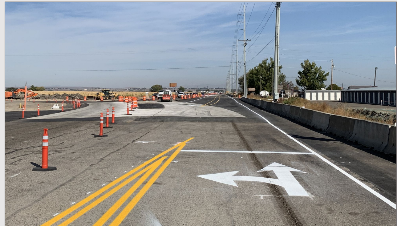
Construction in Progress
