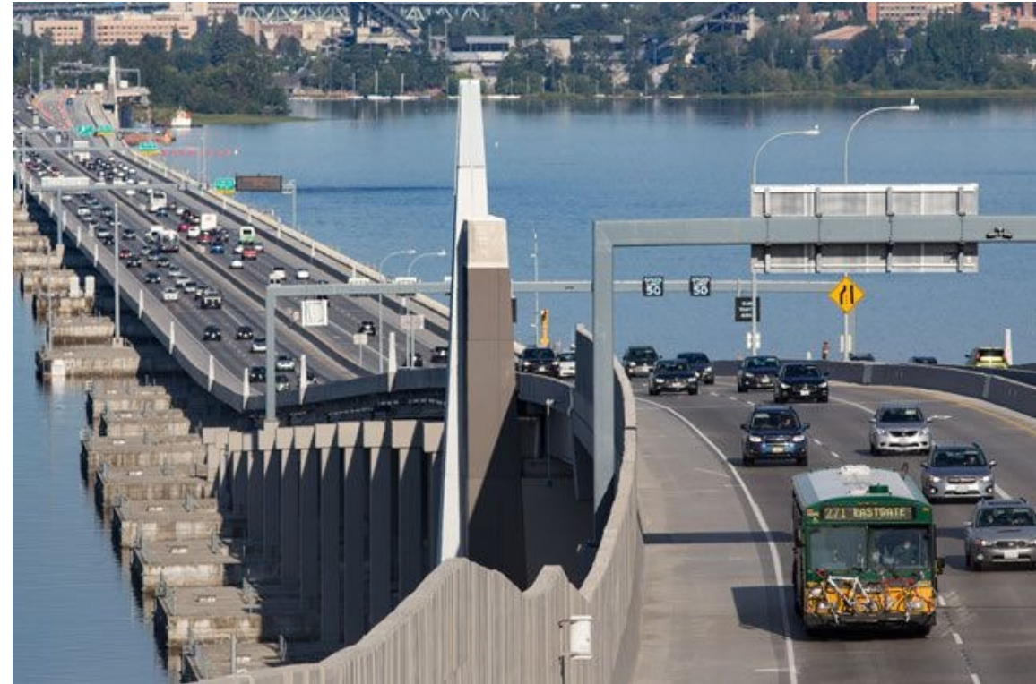
Seattle SR 520 Bridge Source: KIRO 7 News
