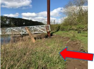
This land (30 feet) has now almost completely eroded. In prior years, this land would flood during winter/spring, but there was no riverbank erosion as illustrated in the next slide. Gangway had to be lowered 3 feet & additional ramp had to be added to gangway for access.
