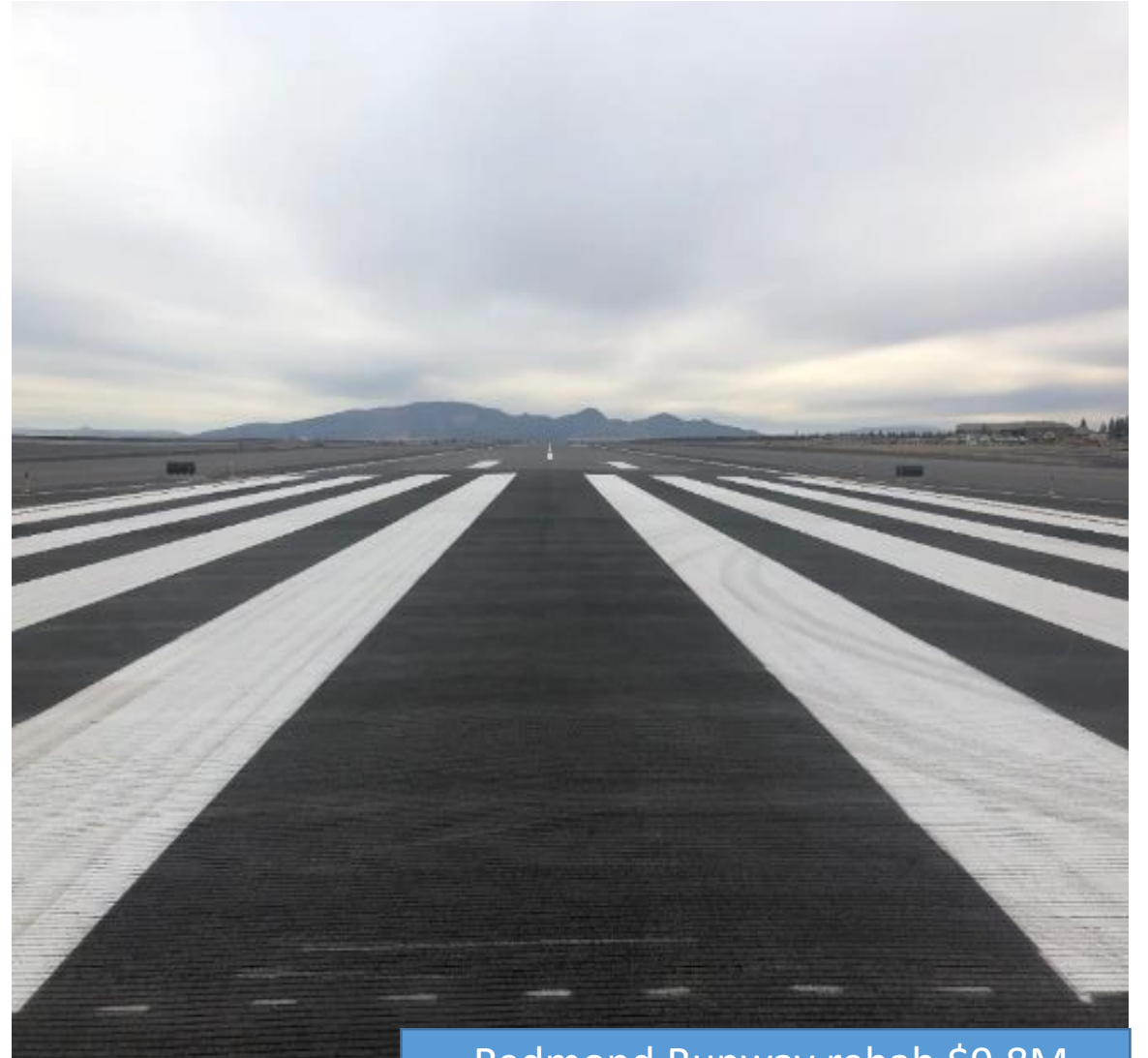
Redmond Runway rehab $9.8M
