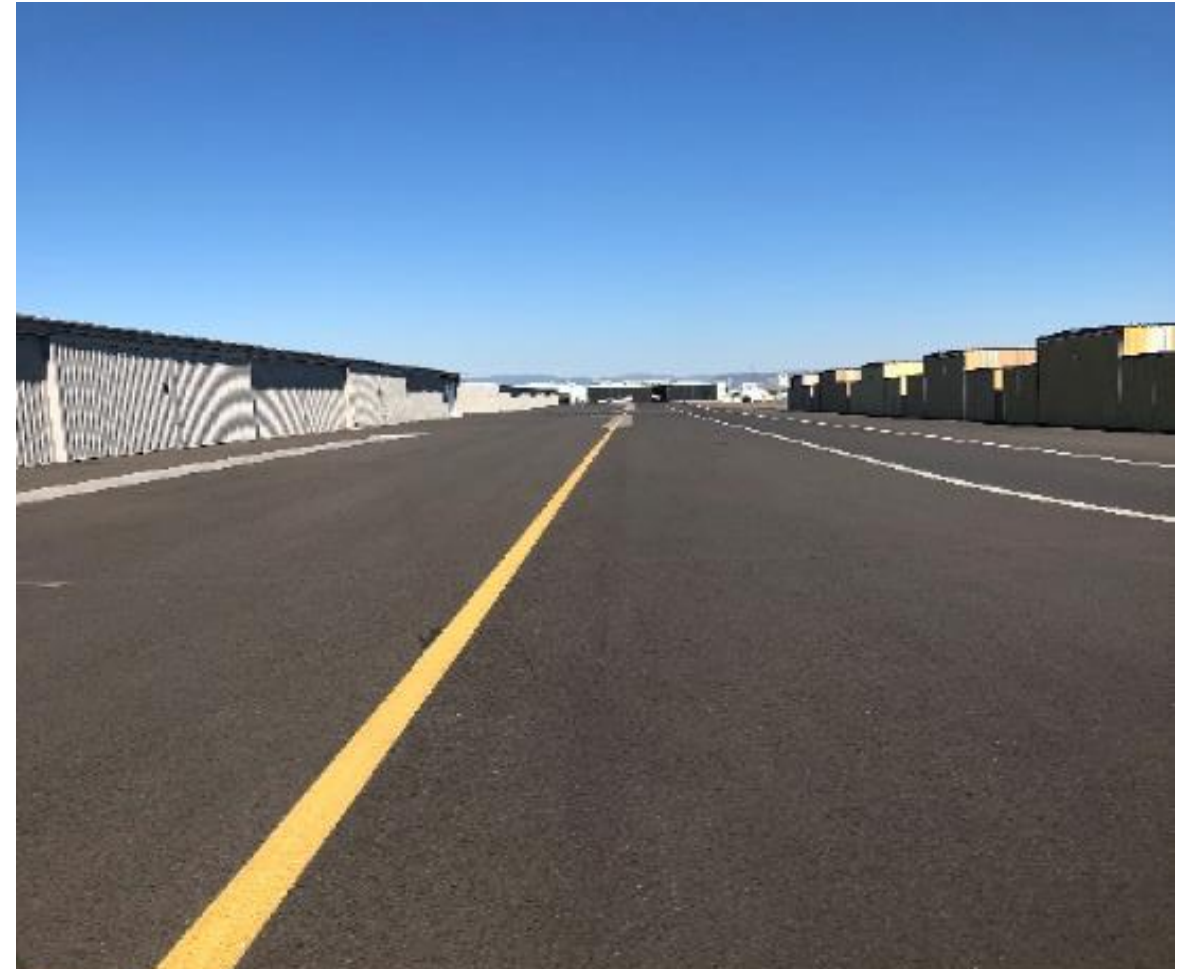
Rogue Valley/Medford general aviation taxiway rehab
