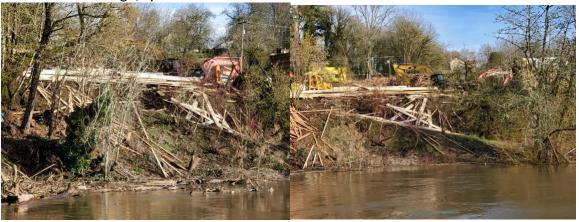
The next photo shows how close the train track runs right ontop of the riverbank for the majority of the 6.5 miles on the Willamette river above the falls heading west. The riverbank's integrity is critical to the structural integrity of the train tracks. You will see a great deal of erosion that is happening along stretches of the train tracks which is causing the residents in this area great concern.
