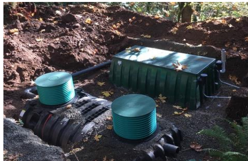
Residential septic system replacement project
