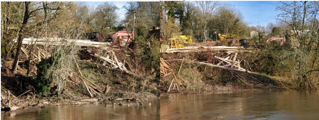
The following photo shows how the riverbank's integrity is critical to the integrity of the train tracks as the riverbank is the foundation for the track.
