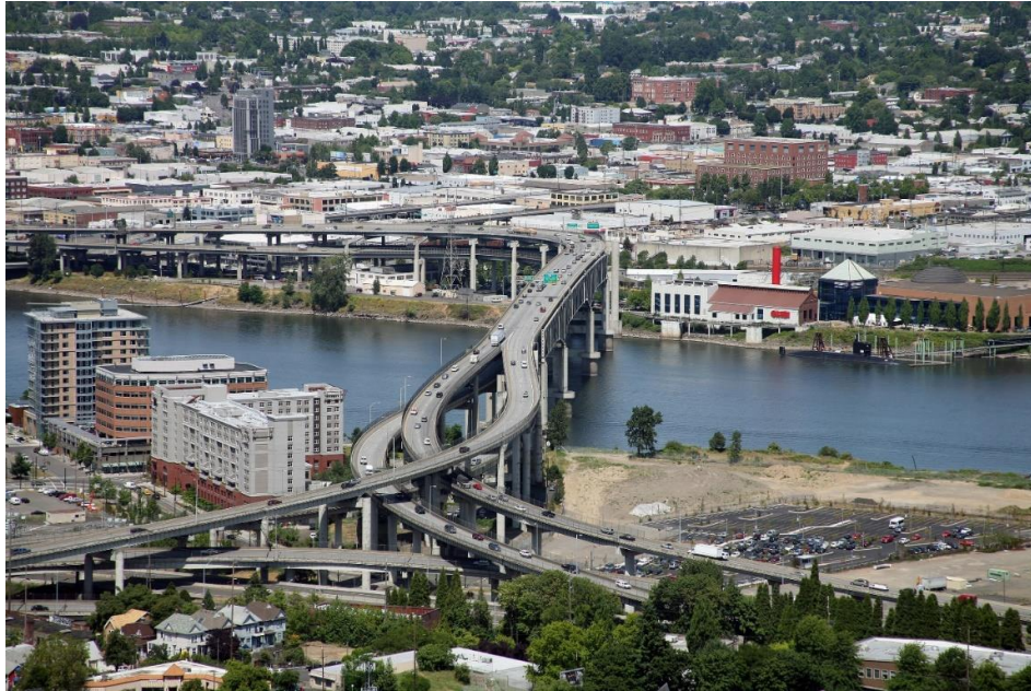
Marquam Bridge, Portland OR
