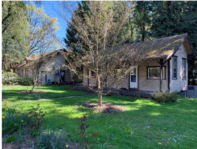
Clackamas Complex Buildings 5 and 6 Currently used by Columbia River Program.
