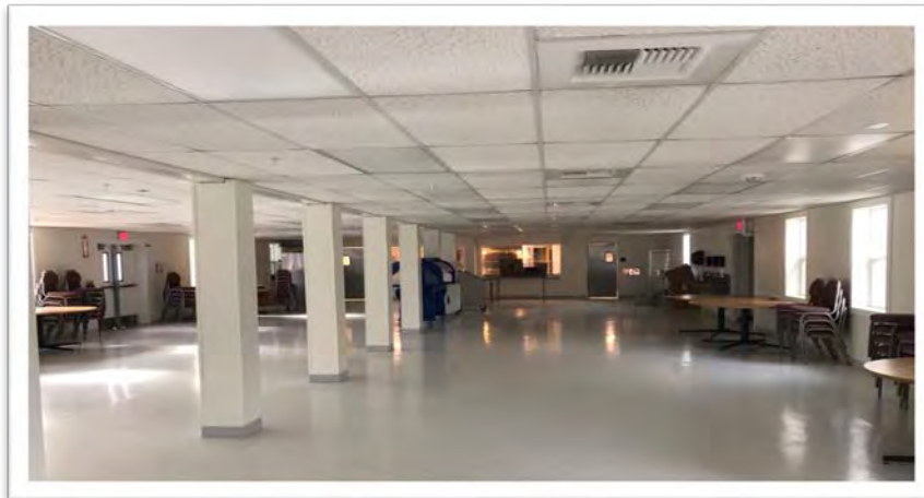
Dining Facility renovation
