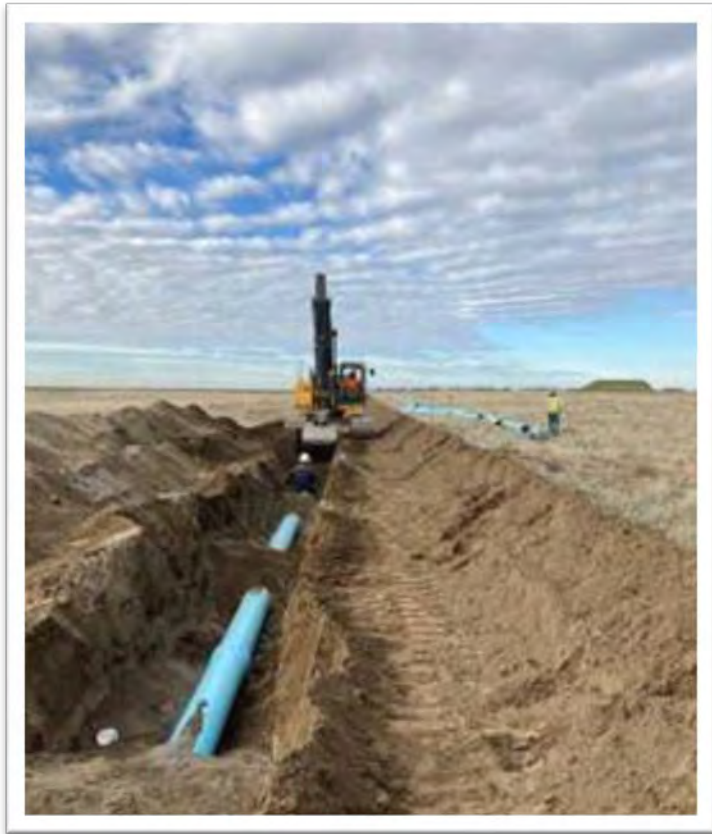
Camp Umatilla Water Line project
