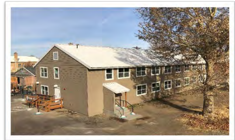
Bldg 5030 Barracks renovation
