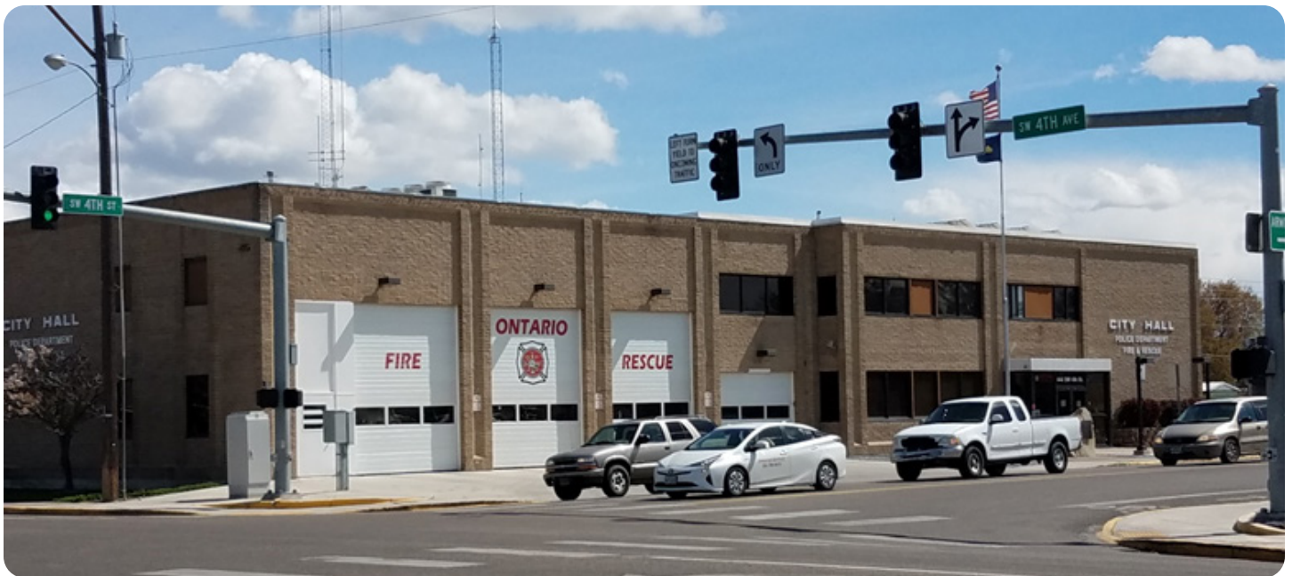
Ontario, Oregon Fire Station. Apr 2018. Photo credit: Tricia Sears
