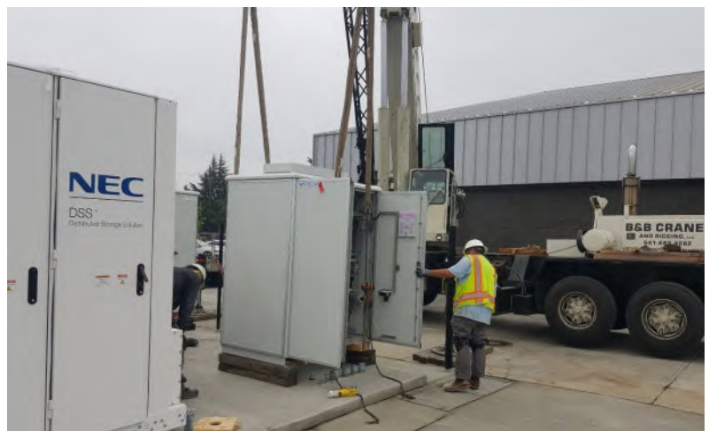
EWEB contractor installs back-up battery power system.
