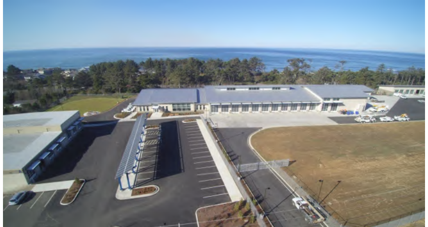
Central Lincoln PUD’s Northern Operations Center, completed in 2017.
