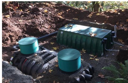
Residential septic system replacement project
