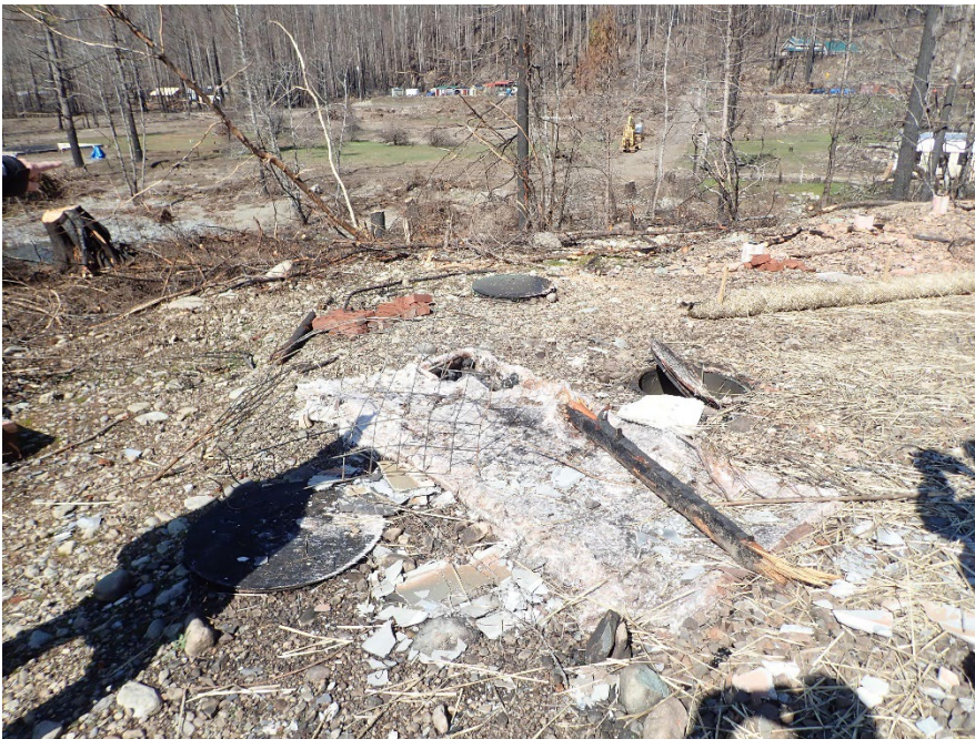
Burned septic system – Detroit Fire, Marion County
