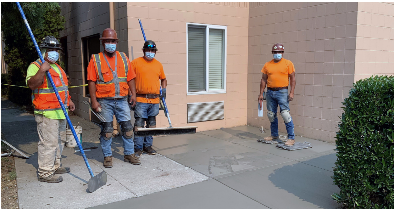
Photo: Oregon State Building and Construction Trades Council (OSBCTC)
