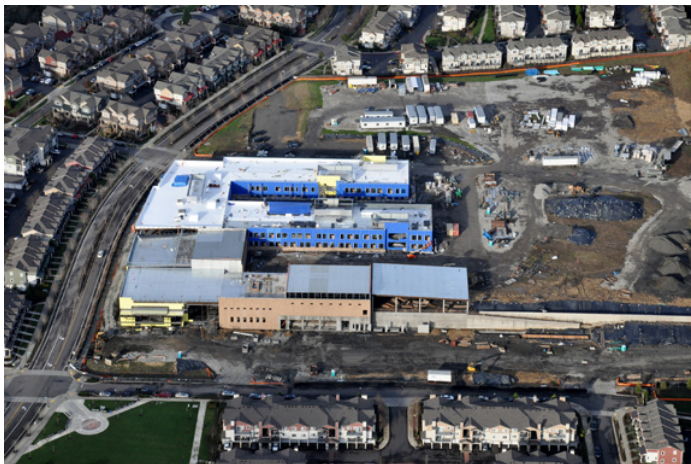
Middle School Aerial View – 12/30/15 (Courtesy BSD)
