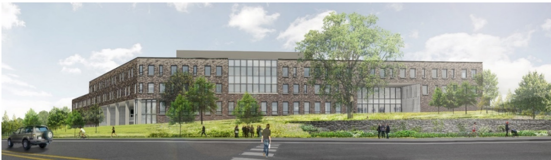
High School at South Cooper Mountain
