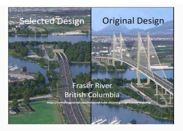
Bridges were originally designed for both the Fraser River and the Fehmarn Baltic Sea crossing. However, after a second analysis by international immersed tunnel engineers, tunnels are now being built.
