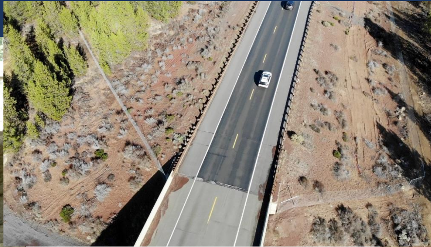
Gilchrist on US 97 Completed 2020
