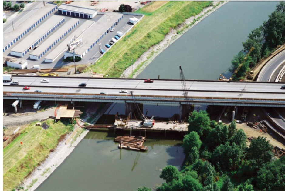
An aerial view of the work bridge with cranes in place.
