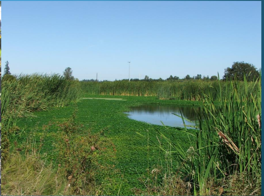
Salem—Wetland Treatment Facility (wet weather treatment)
