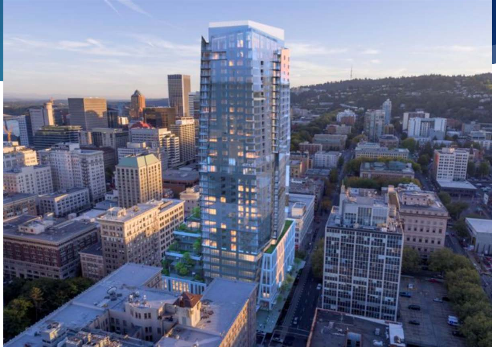
Ritz Carlton under construction, BPM Real Estate Group, Portland
