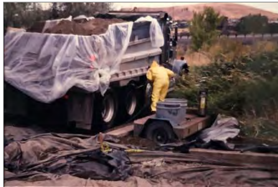
Workers in 1992 removed tons of soil contaminated by the rail tie plant at what is now the city's Riverfront Park.
