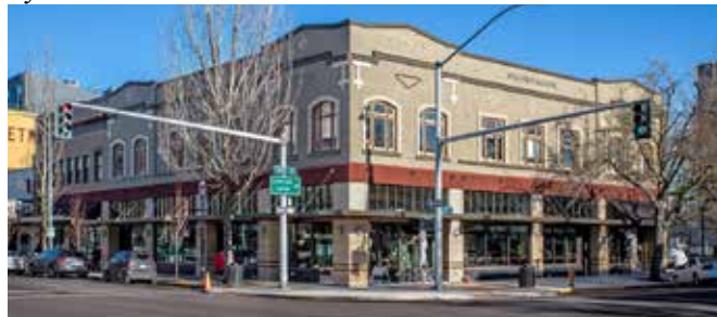
Roth McGilchrist Building, Salem
