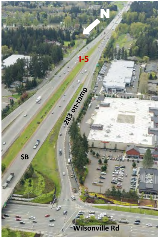
FIGURE 4. I-5 and the Wilsonville Road (Exit 283) south-bound on-ramp.
