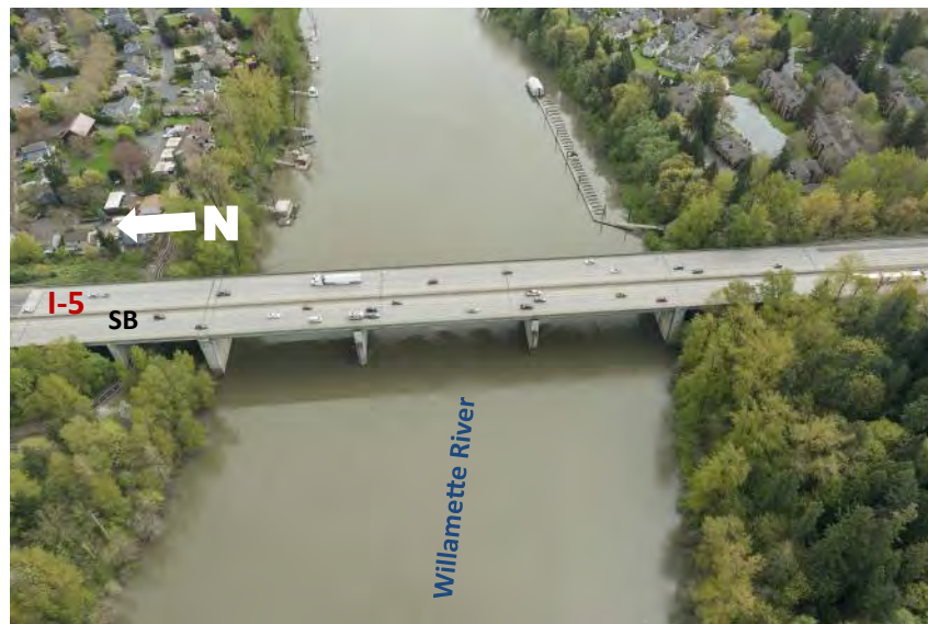
FIGURE 5. I-5 Boone Bridge over the Willamette River.
