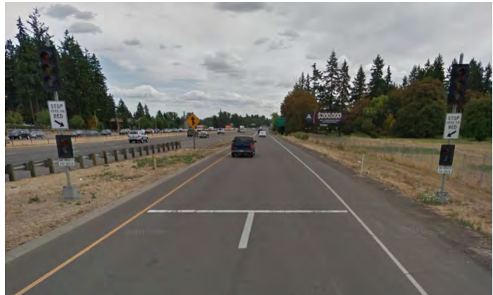
Figure 16: Signal Meter on I-5 Southbound Ramp at SW Wilsonville Road Interchange
